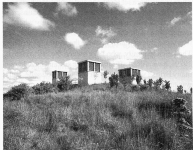
The ventilation towers above the Skendleby RGHQ.
